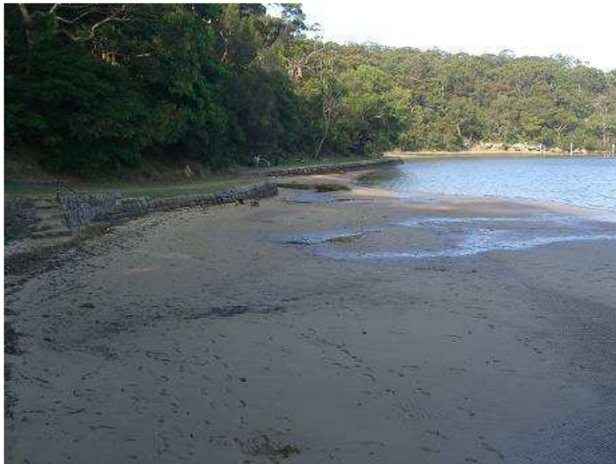
Figure 7.34 – Seawall at Jewfish Bay Swimming Area
