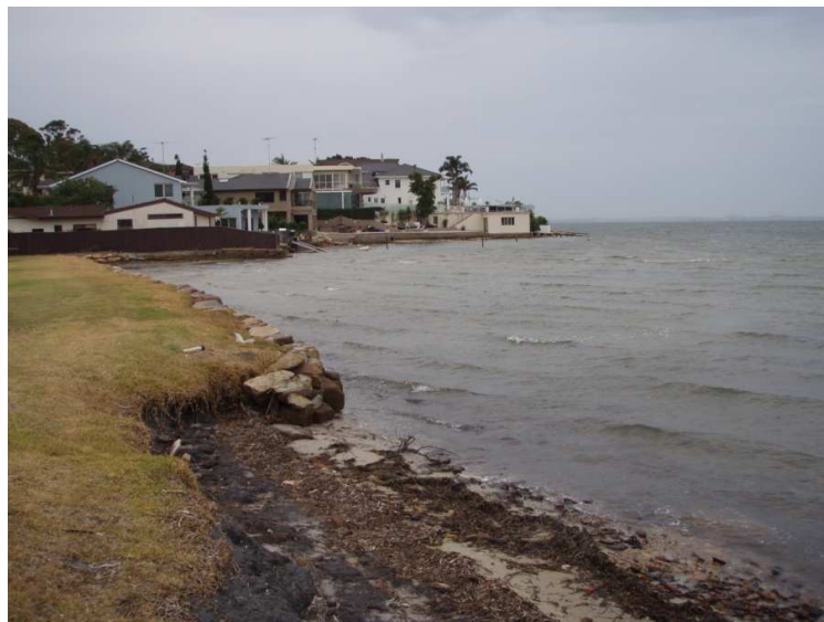
Figure 7.41 – Erosion due to edge effect of a small seawall along the north-western side of Woolooware Bay
