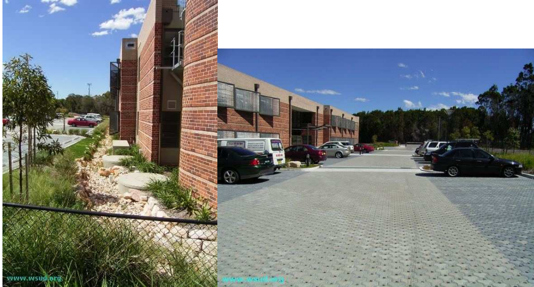
Figure 7.70 – Bioretention along a building and carpark (Left) and permeable paving (right) in Sutherland LGA
