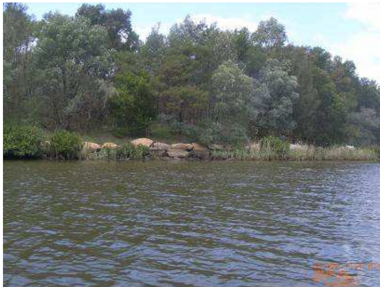
Figure 7.11 – Rock seawall at Howard Park
