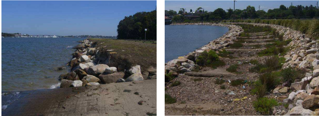
Figure 7.54 – Moderate erosion along low bank at Dover Park (left) and possible solution* e.g. Claydon Reserve at Kogarah bay (right)
