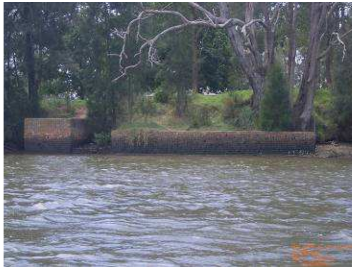
Figure 7.61 – Abandoned brick wall, east of Prospect Creek Mouth
