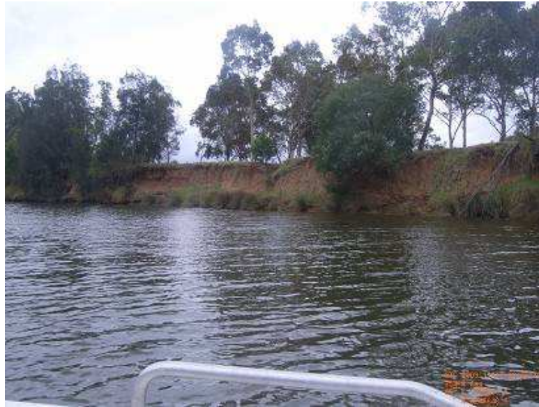
Figure 7.5 – Erosion along Warwick Farm
