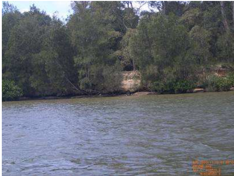
Figure 7.12 – Severe erosion behind vegetation, south of Beatty Reserve
