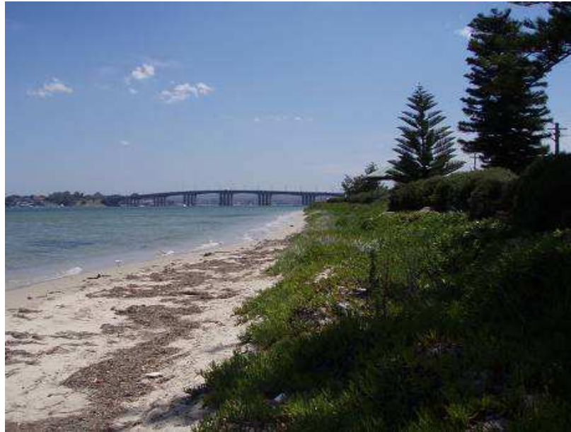
Figure 7.43 – Seawall covered by sand and vegetation east of Captain Cook Bridge
