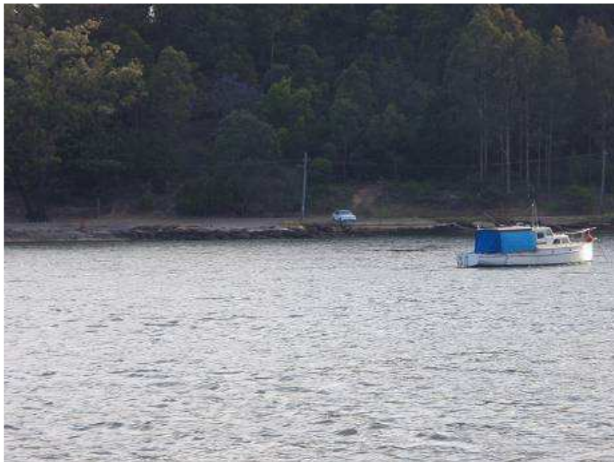
Figure 7.33 – Small rock seawall at Illawong opposite Lugarno
