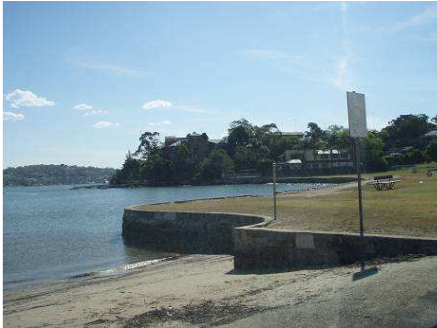
Figure 7.38 – Seawall at Donnelly Park
