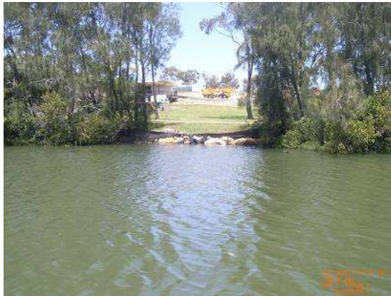
Figure 7.25 – Dumped rocks in gap of vegetation opposite East Hills Park
