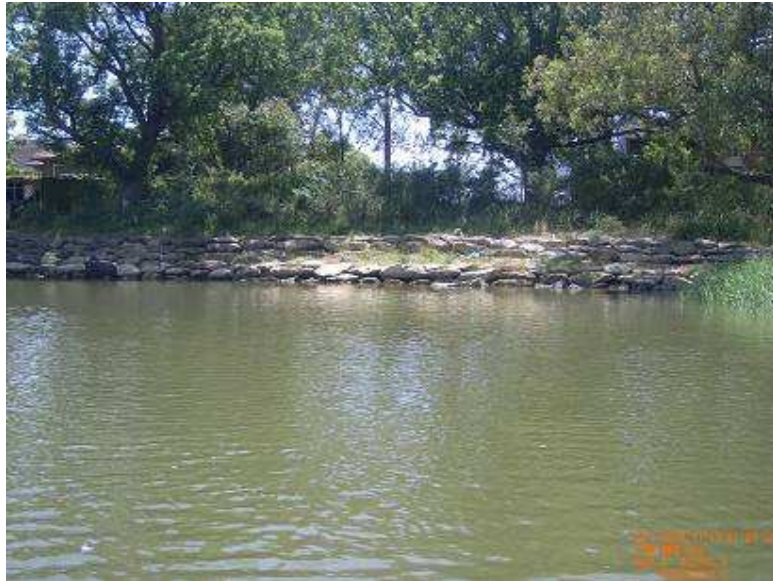
Figure 7.19 – Good condition seawall along Hind Park
