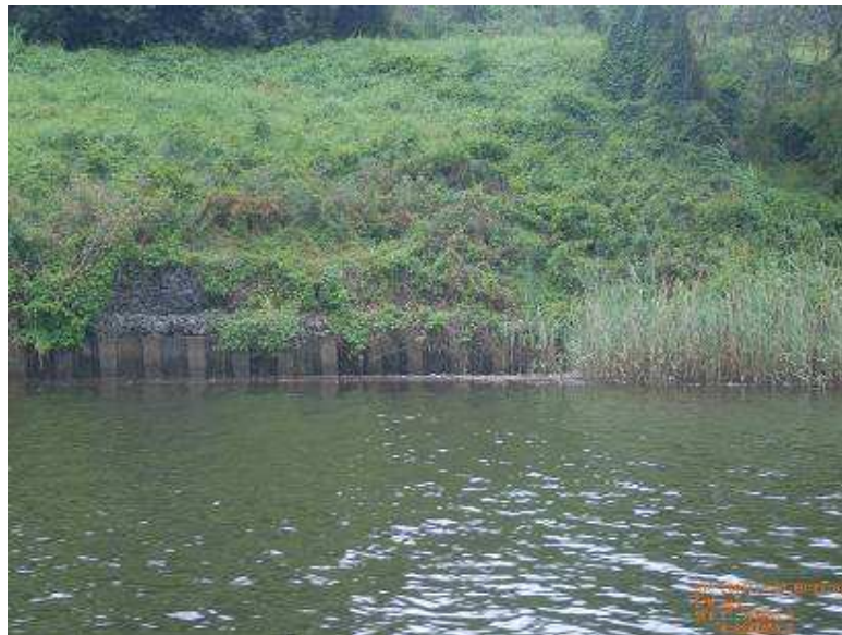
Figure 7.2 – Gabions seawall between McMillan Park and Gandangara Island
