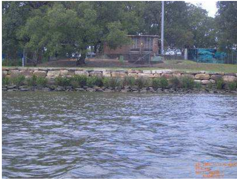
Figure 7.15 – Rock seawall at the northern end of Georges River Golf Course
