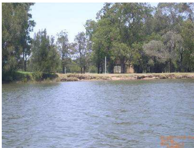
Figure 7.20 – Undercutting along Gordon Parker Reserve
