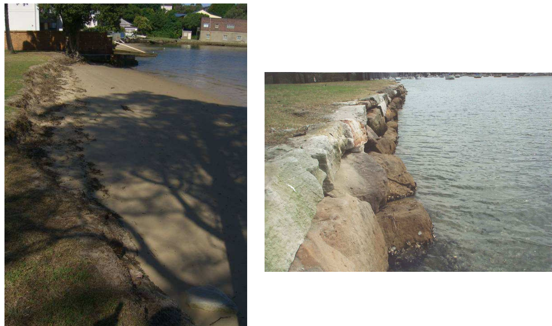
Figure 7.55 – Moderate erosion along low bank at Connells Point Reserve (left) and possible solution** from the DECCW, 2009 (right)
