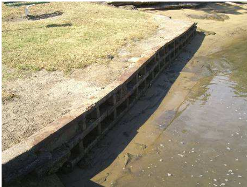
Figure 7.36 – Seawall at Moore Reserve Boat Ramp
