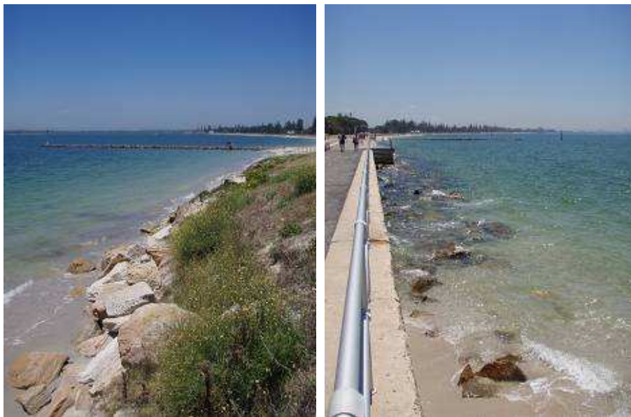
Figure 7.47– Rock seawall in the middle of Lady Robinsons Beach (left) and seawall covered by water at the southern end of the beach (right)
