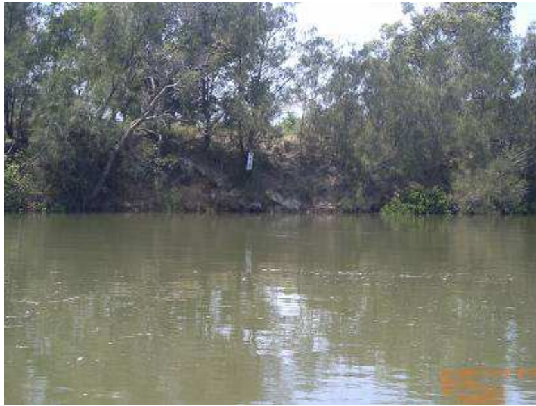
Figure 7.16 – Erosion north of Newbridge Road Bridge, eastern bank
