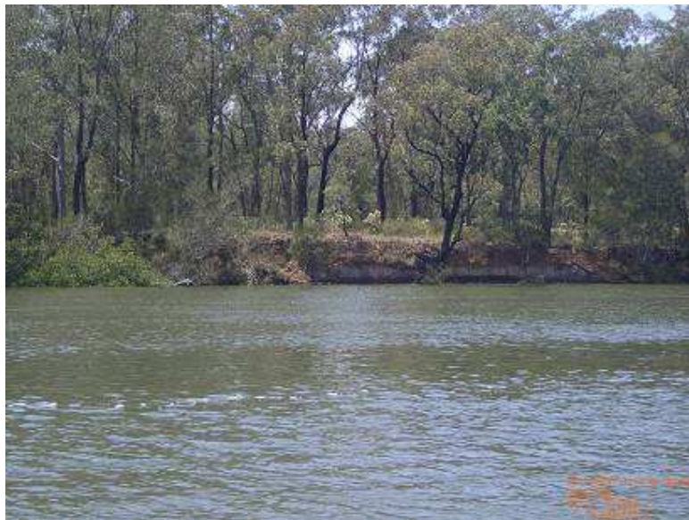
Figure 7.22 – Erosion opposite Williams Creek Entrance
