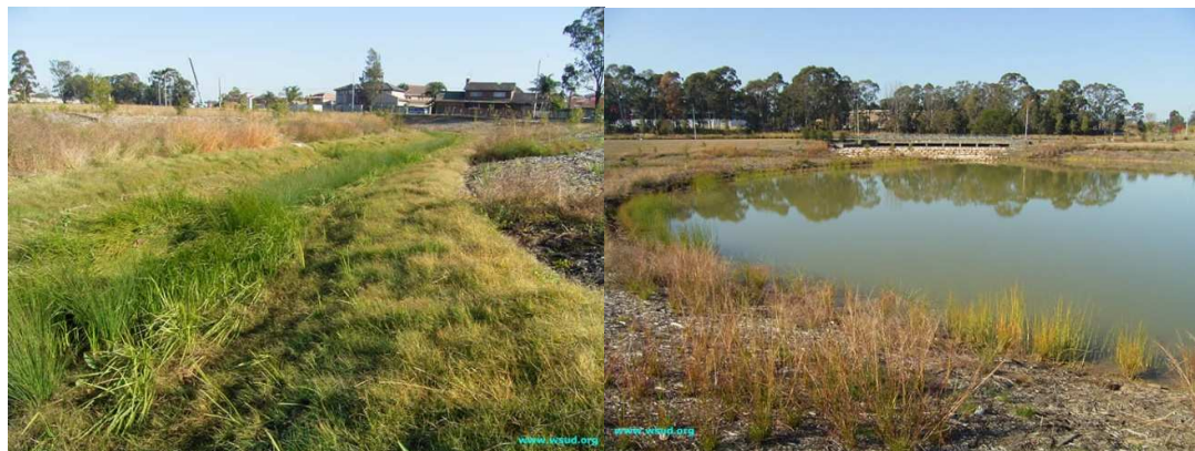
Figure 7.72 – Grassed Swale (left) and constructed wetland (right) in Fairfield LGA
