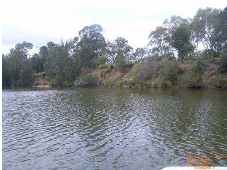
Figure 7.4 – Erosion east of Chauvel Park
