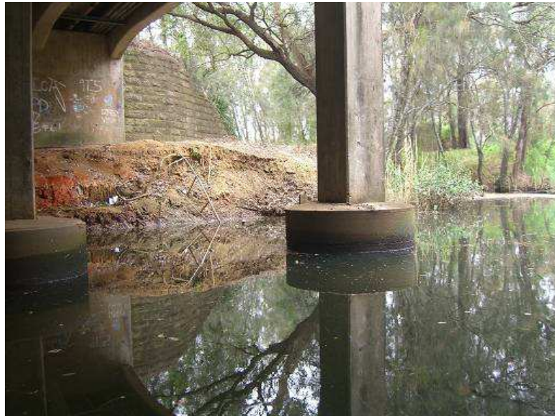
Figure 7.7 – Erosion under Hume Highway Bridge
