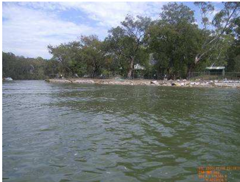
Figure 7.28 – Seawall maintenance along Picnic Point
