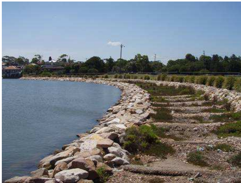
Figure 7.42 – Good condition seawall at Claydon Reserve, Kogarah Bay
