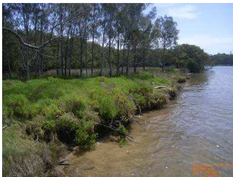
Figure 7.32 – Light undercutting opposite Little Salt Pan Creek
