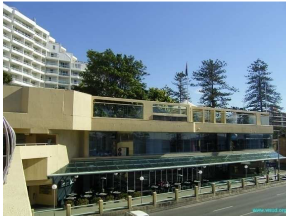
Figure 7.74 – Greenroof at Brighton Le Sands in Rockdale LGA
