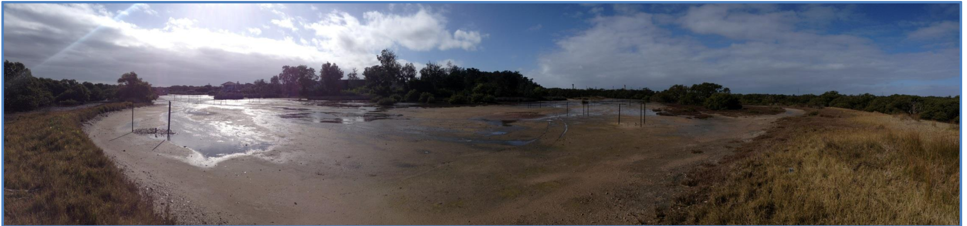
Figure 11. Panoramic photograph of Site. Taken July 2013 after the completion of revegetation works.
