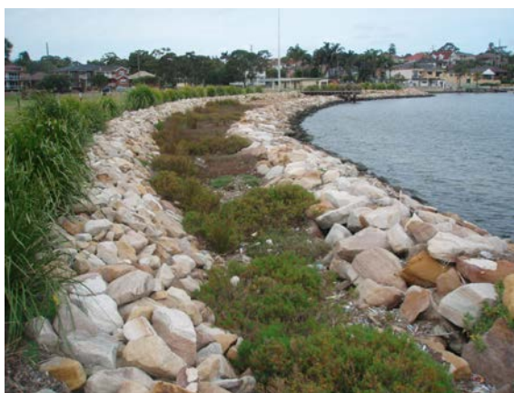
Eco-friendly seawall, Kogarah (photo: OEH)
