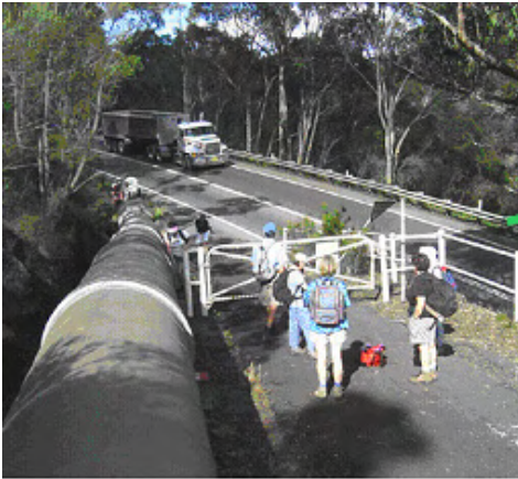
Heathcote Road major arterial highway crossing is currently hazardous
