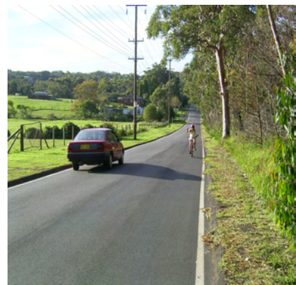
Walker St from Helensburgh to Kellys Falls – no shoulder for 800 m on an 80 km/h speed limit road
