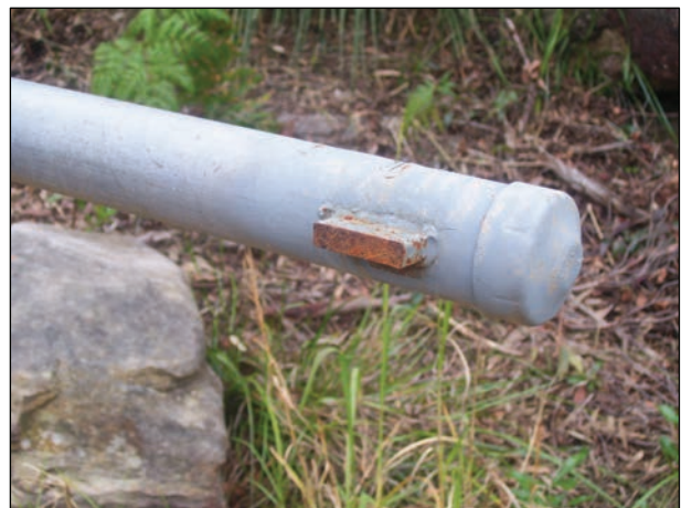
Hacksaw padlock assembly on a light-weight access gate on Treloar Place.
