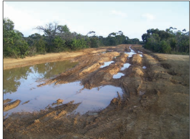
Track widening and ponding, western bushland.
