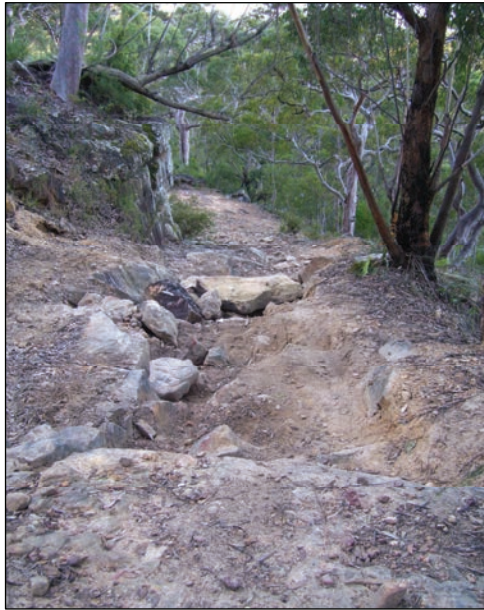
Badly eroded and impassable management access trail.
