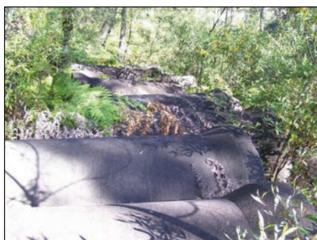
Large reinforced concrete pipes, dumped beside Mill Creek (just north of the old mill site), could be recycled/used as barriers in rationalisation of the vehicle track network.
