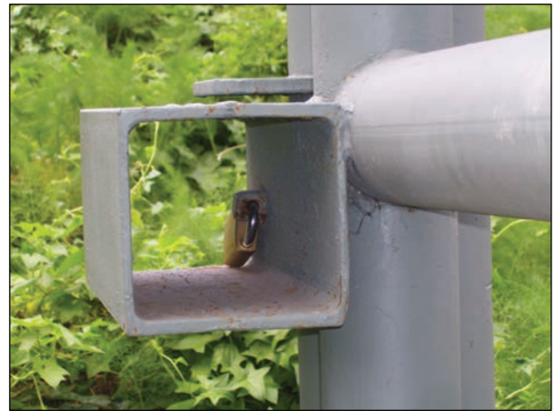
Examples of high security gates and padlock assemblies, from Botany Bay National Park.
