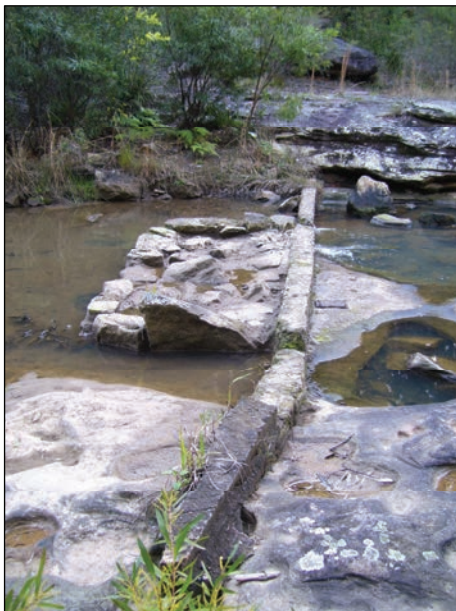
Remains of the Old Flour Mill weir which also serves as an informal creek crossing point.
