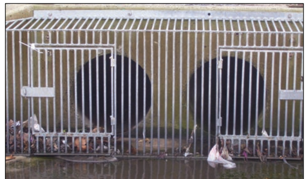
Grates and Gross Pollutant Traps are essential first line stormwater management devices, and necessary to get the best from other secondary measures.
