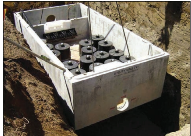
A prefabricated sub-surface sand filter unit, suitable for retrofitting below roads and verges.
