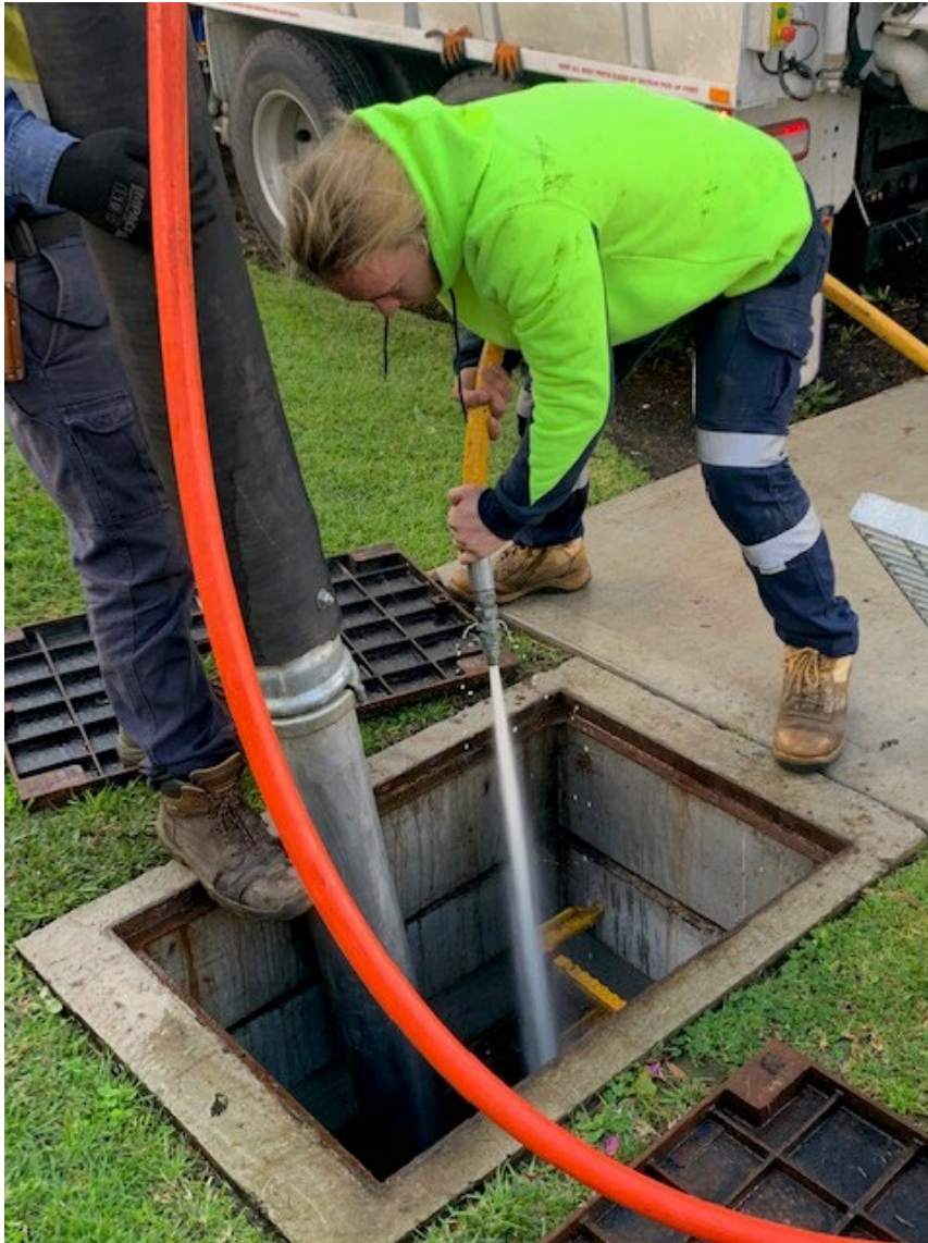
Figure 17 High pressure cleaning of screens and internal areas of the GPT is recommended for every clean.
