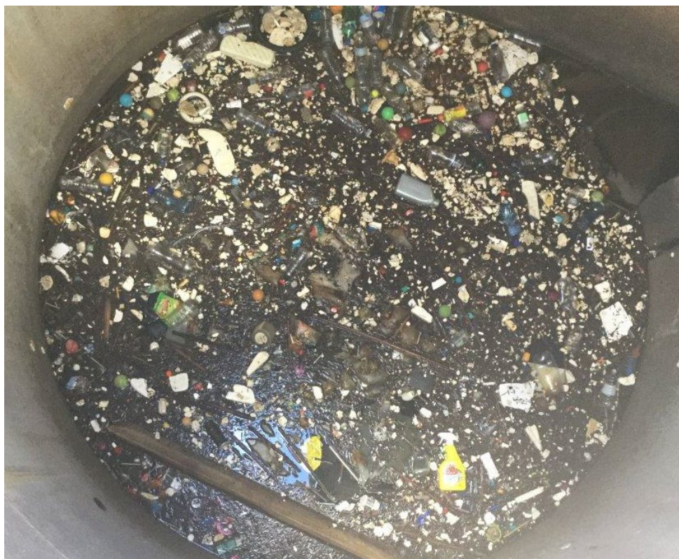
Figure 3 Stormwater pollution trapped in a CDS unit at Fairfield. Without the insurance of GPTs like this one, all of this would have ended up in our creeks, river and ocean. Image c/- Optimal Stormwater 2018.
