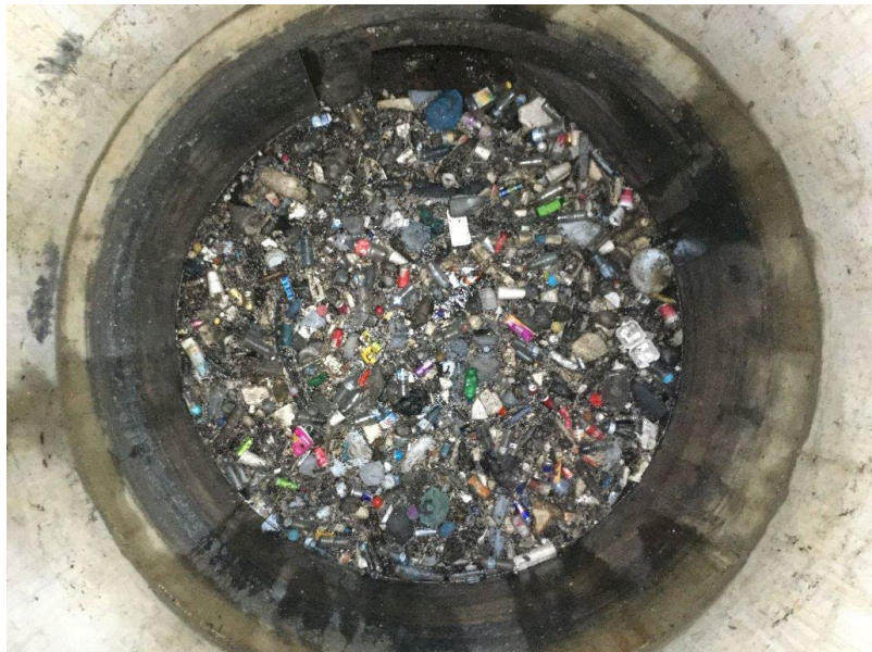
Figure 2 Stormwater in a CDS unit. 3% floats and that's what's seen here, but 97% will waterlog and sink, needs to be cleaned from the sump below. Image c/- Optimal Stormwater 2018.
